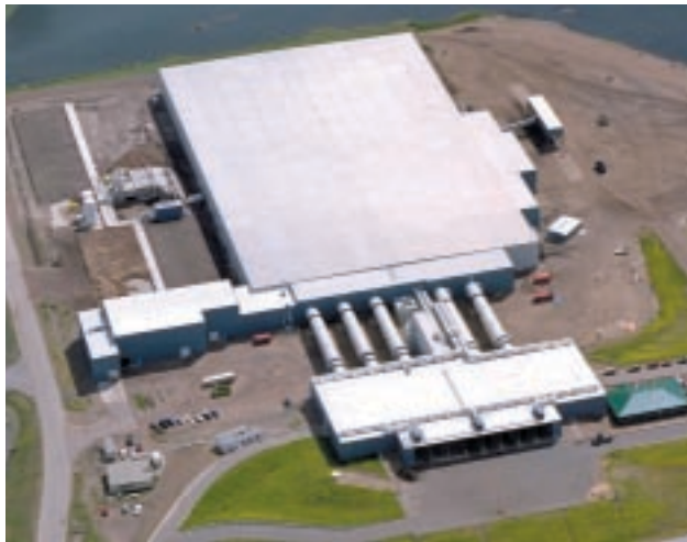
The MBT facility in Edmonton, Alberta
